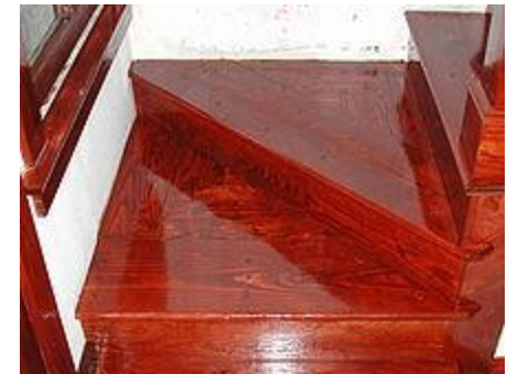
Varnish on wood stairs
